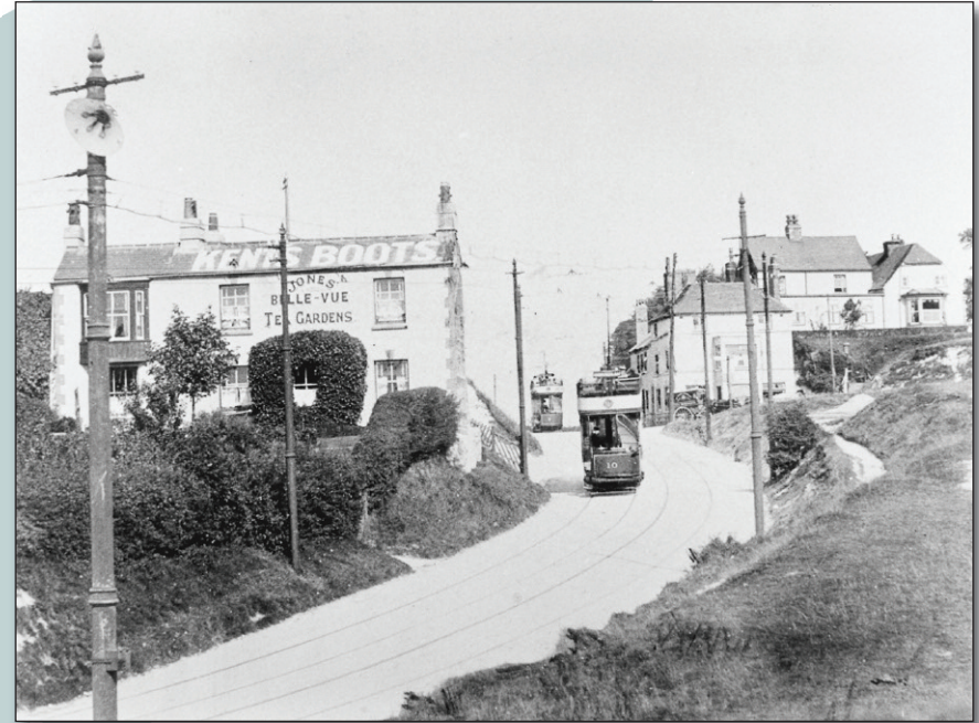
Two trams of the Portsmouth and Horndean Light Railway prepare to pass each other at the crossroads in those quieter days at the beginning of the last century.
